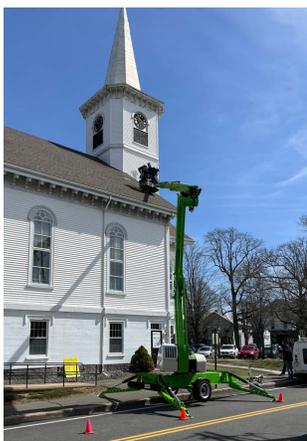
We also coordinated with two contractors to replace the missing shingles on the sanctuary roof that blew off in one of the recent windstorms. An 80 ft. height capacity lift was used to get the roofing repair contractor onto the roof. While on site, we also used the lift for the roofing contractor to replace the two half moon plexiglass tops of two of the tall sanctuary windows on the Church St. side. We have not received a bill for this work yet.
